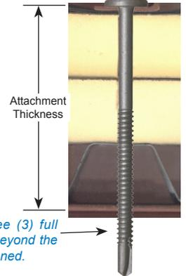
Allow at least three (3) full threads to extend beyond the material being fastened.
